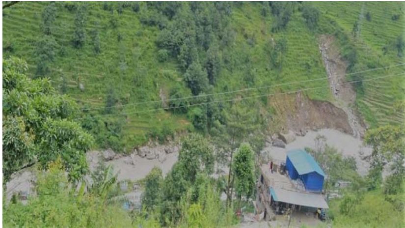
Photograph 1: Power house on construction Phase
