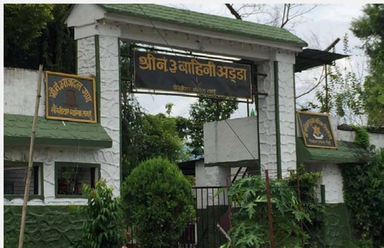
Figure 3.10: Army barrack at Khairenitar bazaar
