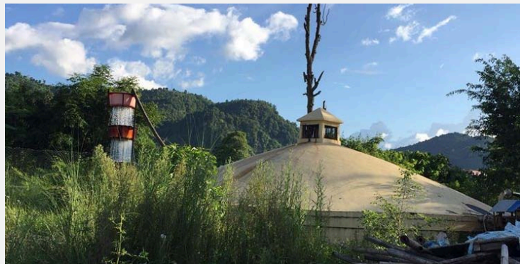
Figure 3.13: Perforated trays for oxidizing iron content in groundwater
