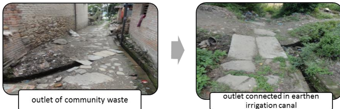
Figure 1: Channelling of wastewater for irrigation purpose
