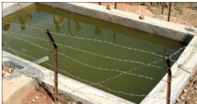
Figure 11: Water harvesting concrete pond
